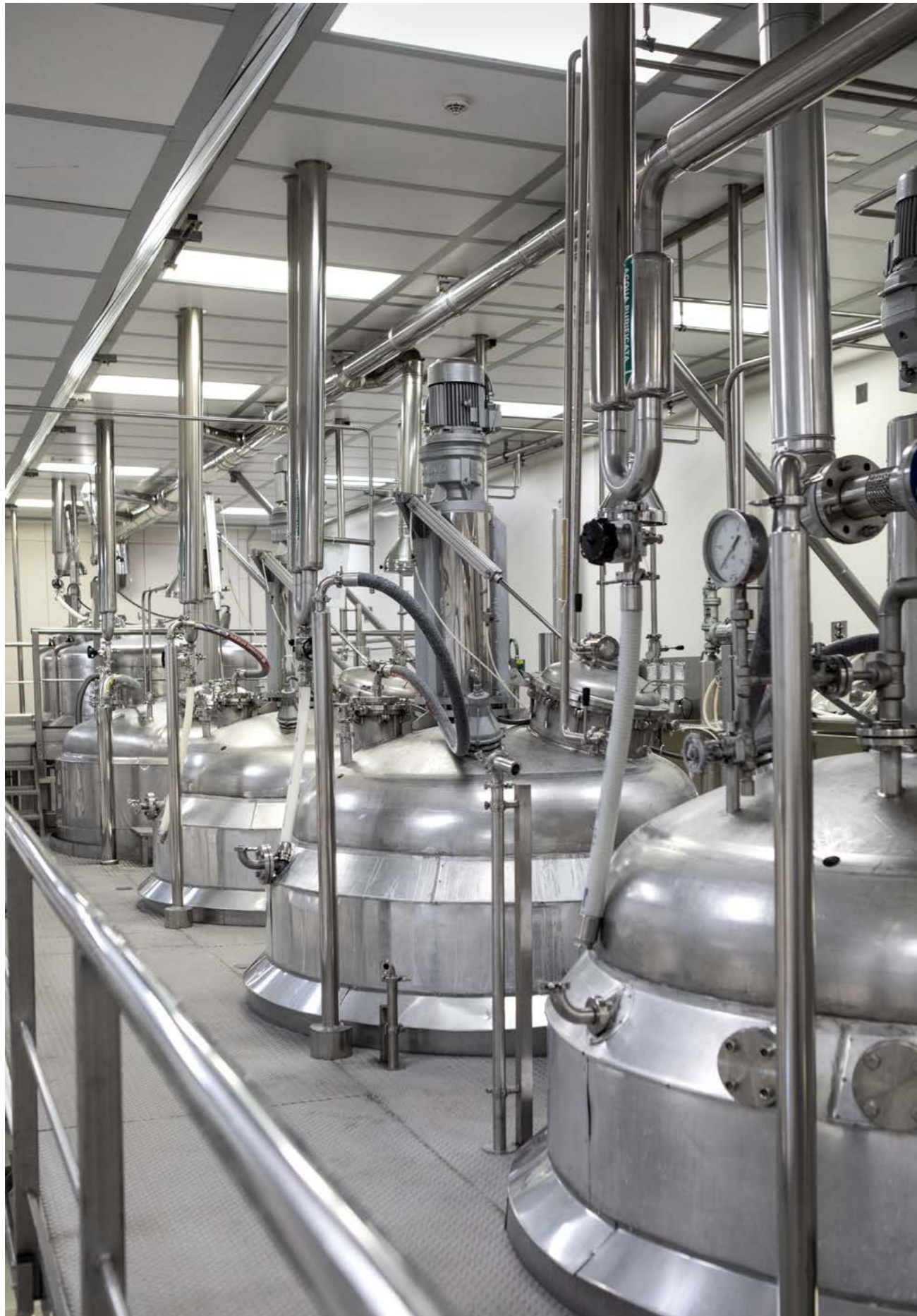
Inside the Ancona plant
